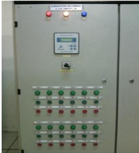
**Gambar 3** Panel Capacitor bank
